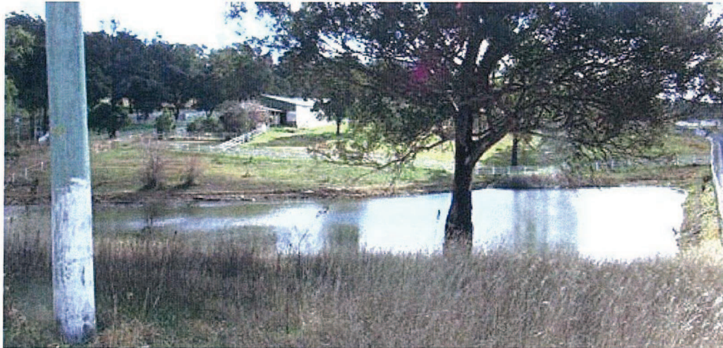
Photo 8 – Eastern end of the largest dam.
